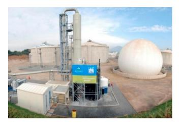
**Figure 12**: Biogas production and upgrading plant in LaFarfana, Chile (*Source: NGV Journal*)
